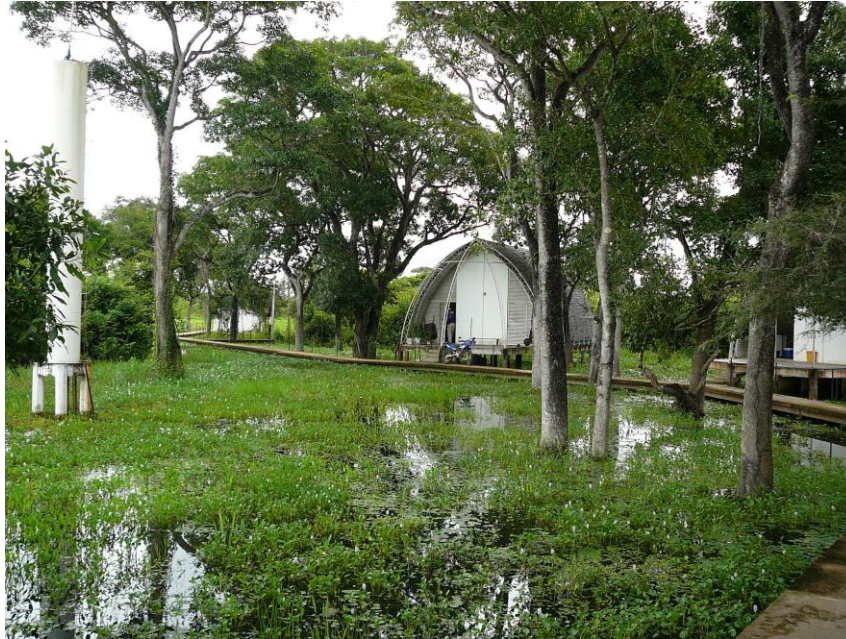
UFMT's advanced Research Base in the Pantanal. Accommodation for 20 people, including laboratory, classroom, dormitory, cafeteria along with access road throughout the year
